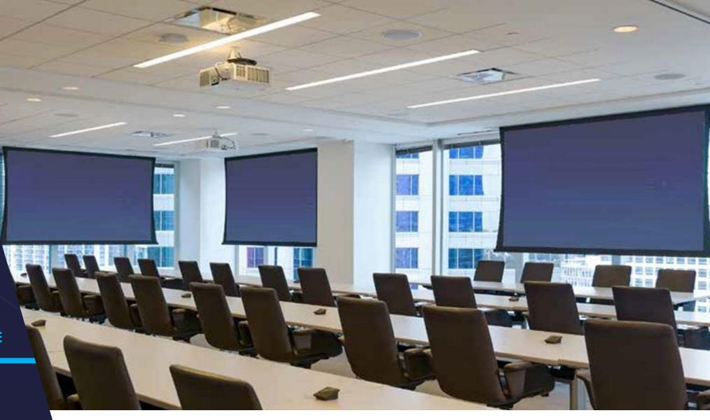
The Seyfarth Shaw triple divide/combine meeting space features laser projectors, retractable ambient light rejecting screens and pan /tilt/zoom videoconferencing cameras.
